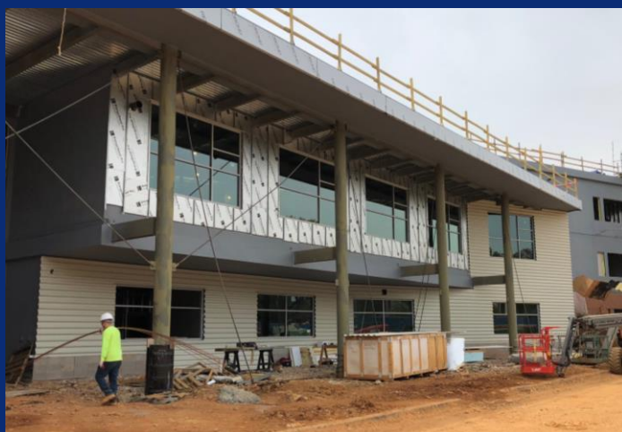
Metal Panel Install at North Entrance (Elevation F)
