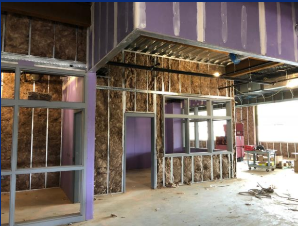
Insulation Install at Second Level Media Center
