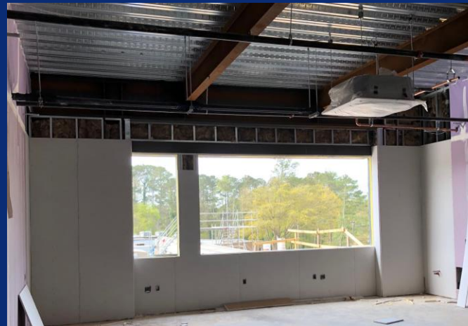
Second Level Classrooms Drywall Install
