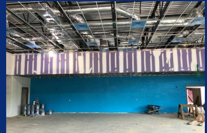
First Coat of Finish Paint in Cafeteria
