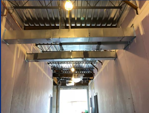
Mechanical Duct Install at Second Level East Corridor
