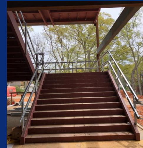
South Stair Installation (to receive precast treads and stainless handrails)
