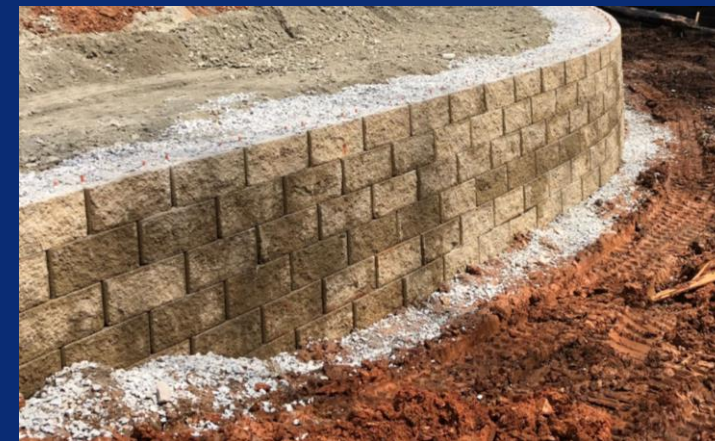
Modular Block Wall Installation
