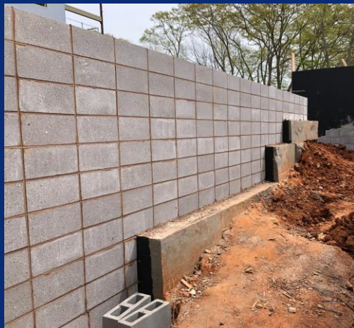
South Entry Ramp/Stair Walls Dampproofing and ACMU Veneer
